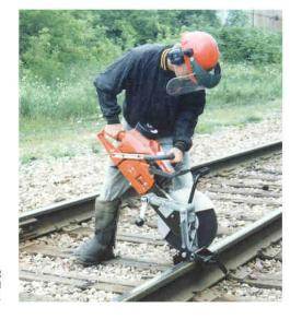
Lightweight 44 lb power unit easily attaches to clamp and arm assembly
